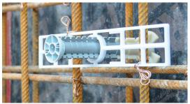
By using fitting plate and extension sleeve, the installation depth and also the guaranteed save working load, will be increased to 4'500 kg (45kN).
