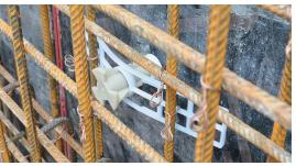
Thanks to the fitting plate, the cone is pressed to the formwork in an optimal way.
