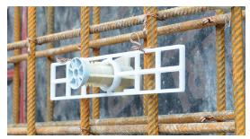
With internal formwork, pillar or steel formwork, tie the fitting plate to the reinforcing rods.
