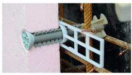
Application of the UNI-concrete sleeve with fitting plate and extension sleeve with inlaid insulation in the formwork.
